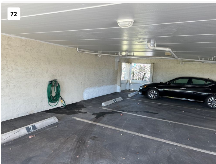
Painting and priming in progress.
