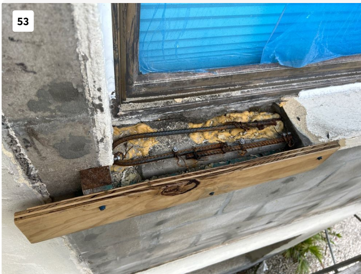
Window sill repair in progress.
