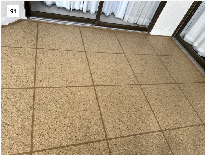
Rear balcony polyurethane waterproofing membrane with gemstone acrylic coating.
