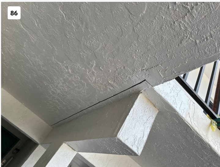
Underside of expansion joint.
