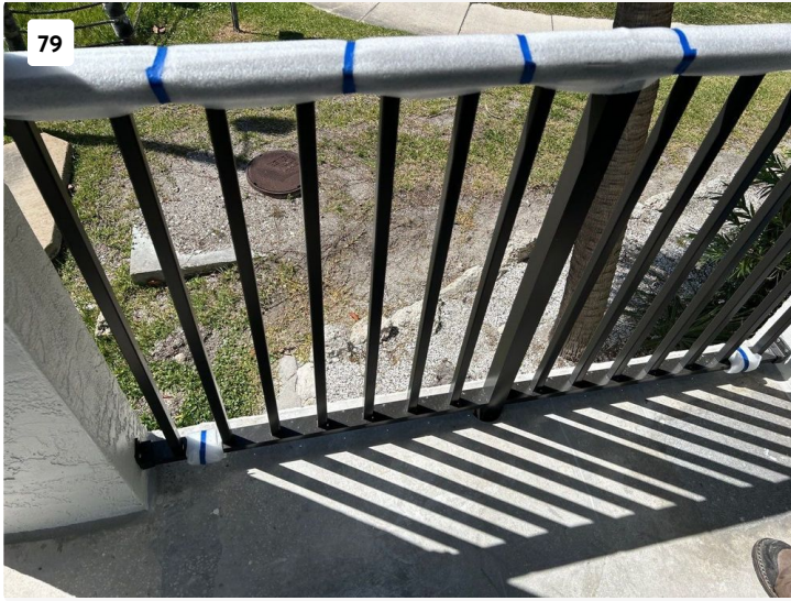
New balcony rail installation.
