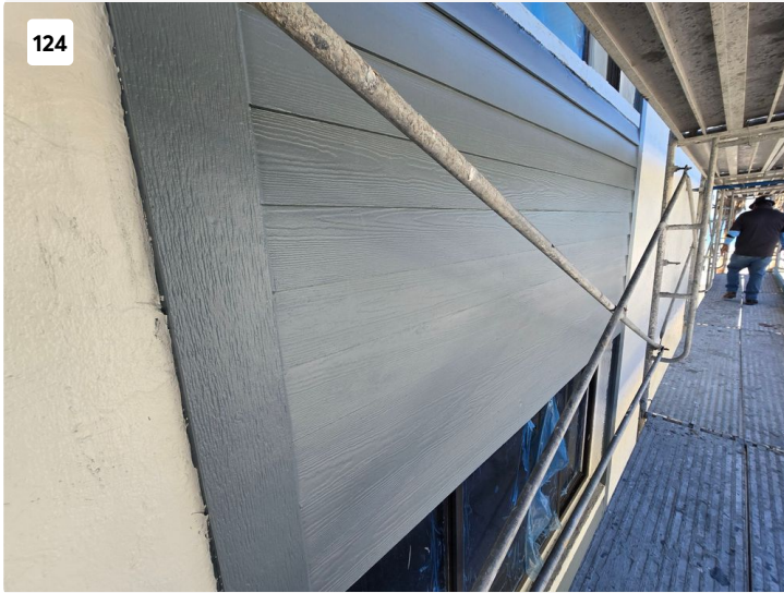
New hardie board trim installed.
