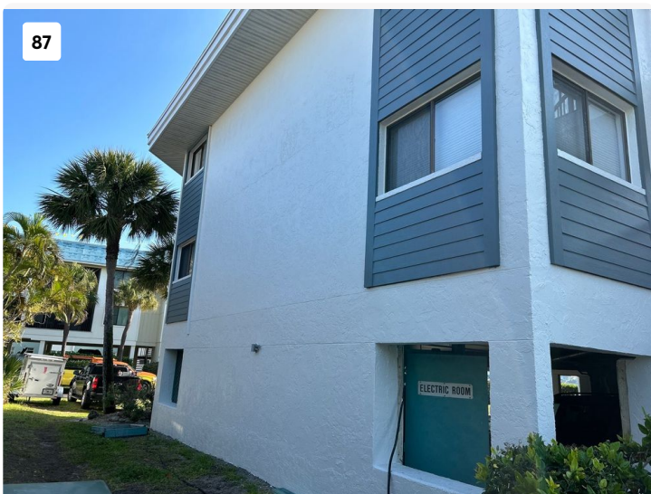
Hardie board trim and exterior painting completed
