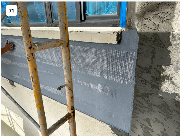
Waterproofing of CMU block in preparation for hardie trim.
