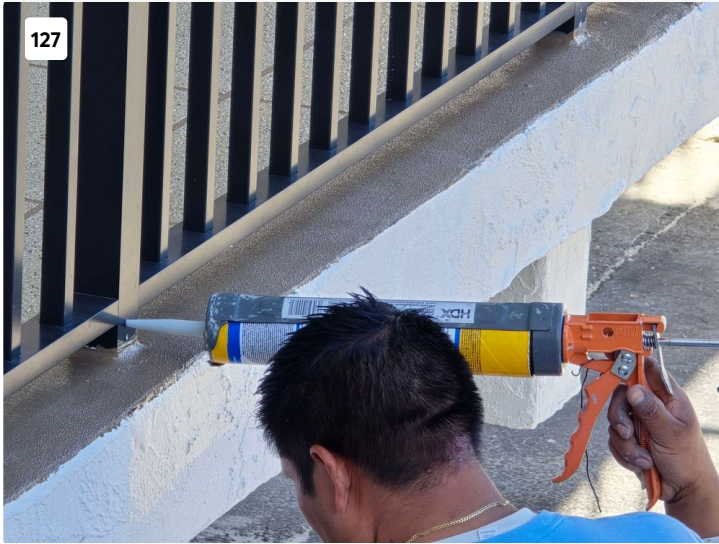
Drill and fill of new rail post.
