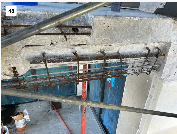
Balcony beam repair in progress.
