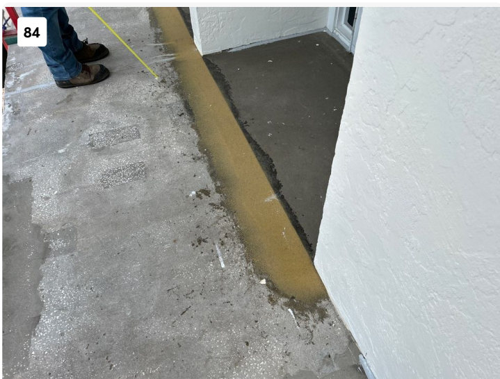
Cementitious and epoxy sloping at entry door.
