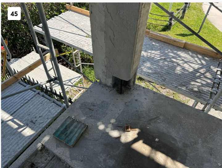
Balcony column spall repair in progress.
