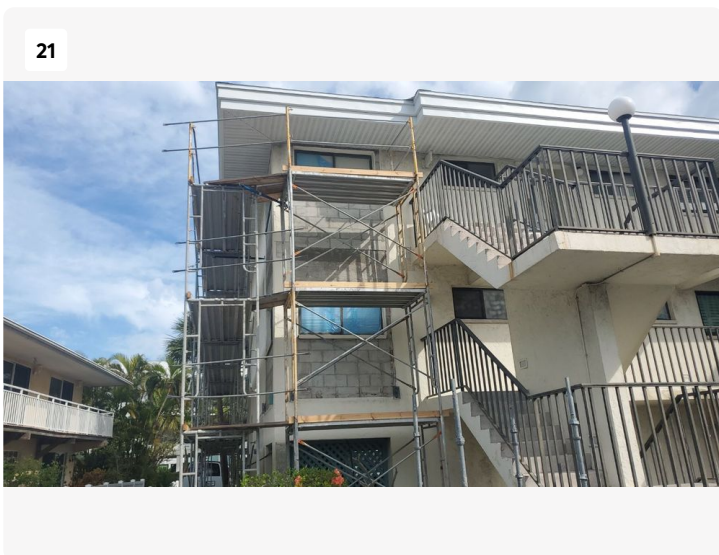
Damaged and rotting wood trim around window opening has been removed.
