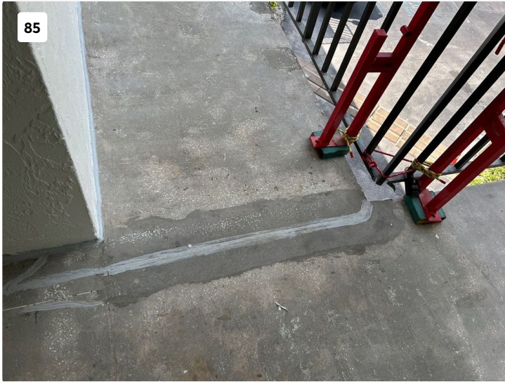
New walkway expansion joint sealant installed.
