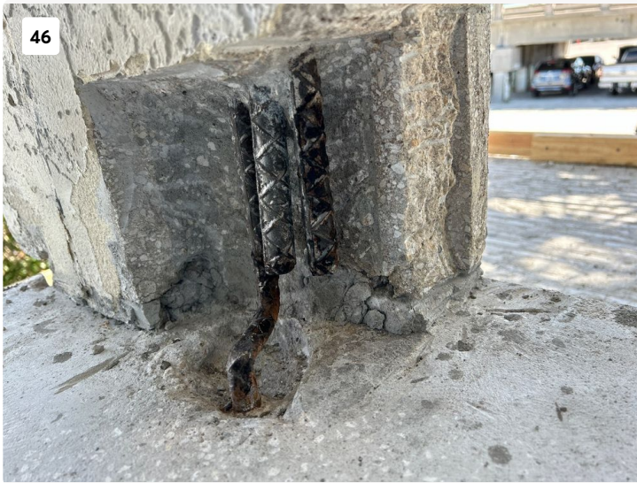
Balcony column spall repair in progress.
