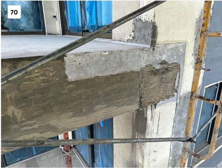
Completed balcony concrete repair.
