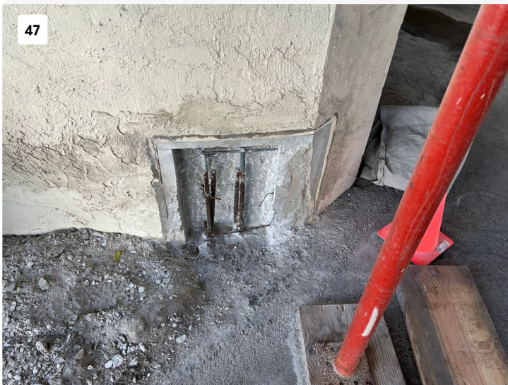
CIP garage column spall repair in progress.
