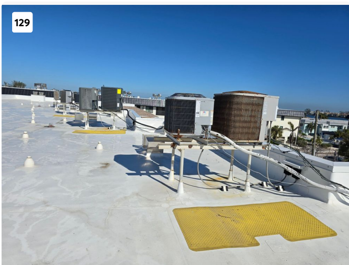
TPO flat roof installed circa 2022.
