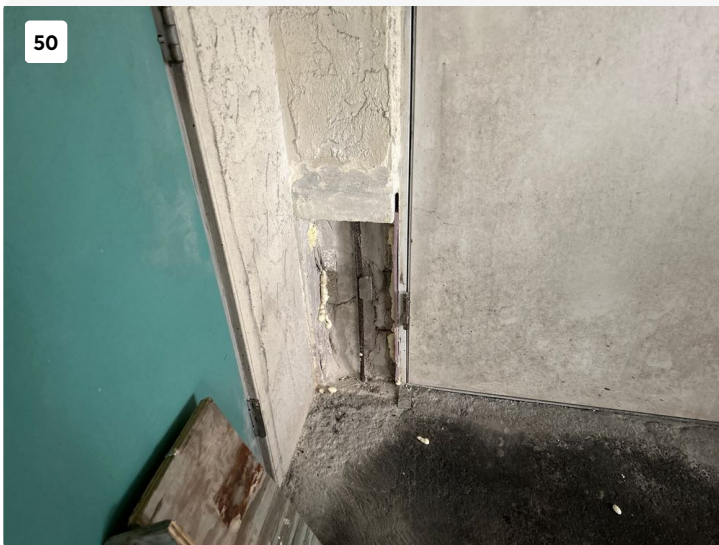
Concrete spall repair in progress. Sacrificial anode placed on reinforcing.
