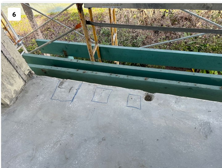
Sounding and marking of balcony deck spalls.
