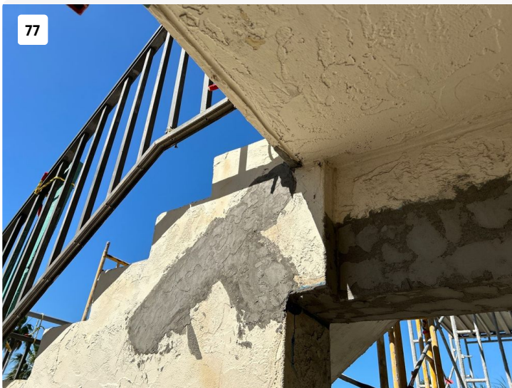
Stucco repair in texture phase.
