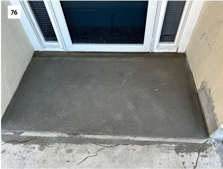
Front entry sloping and crack chasing in progress
