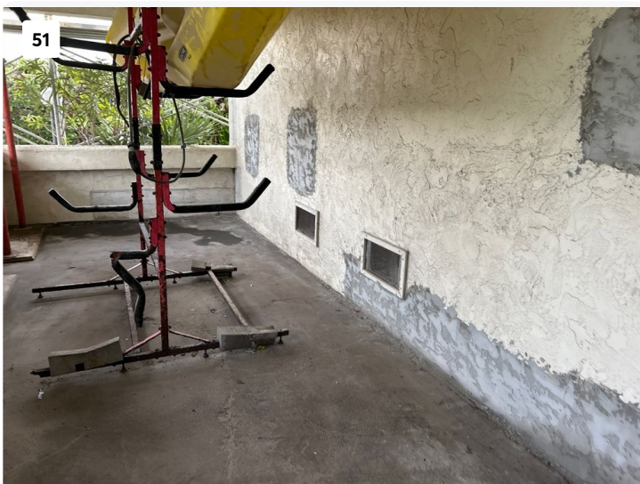
Garage stucco replacement in texture phase.
