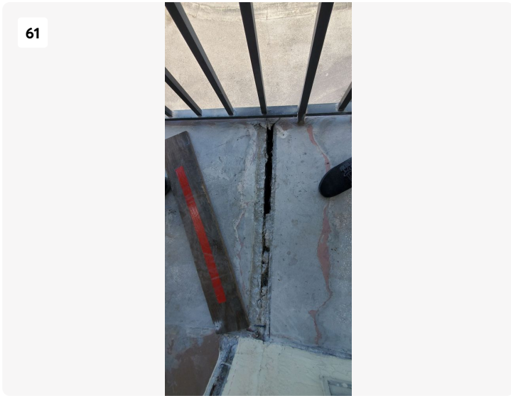
Control joint between hollow cores.
