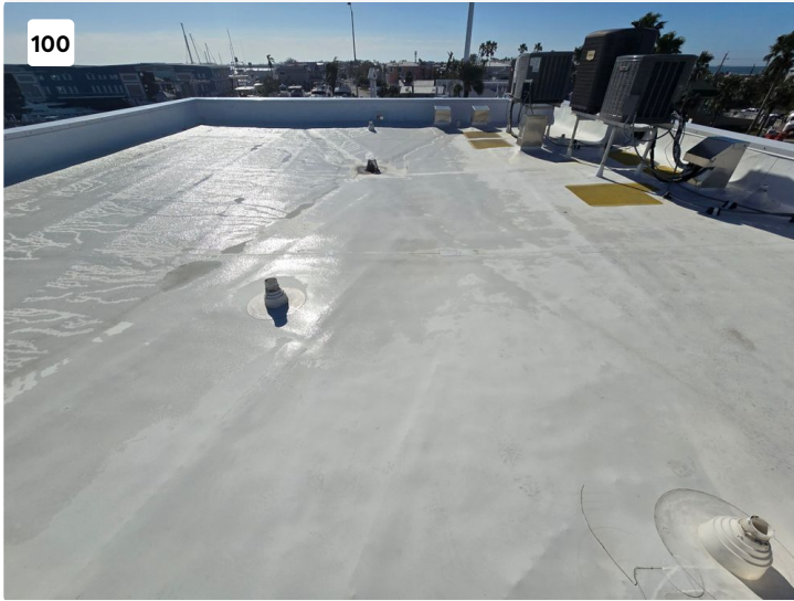
TPO flat roof installed circa 2022.
