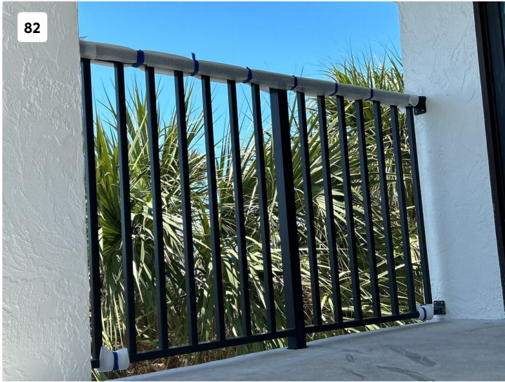
New balcony rail installation.
