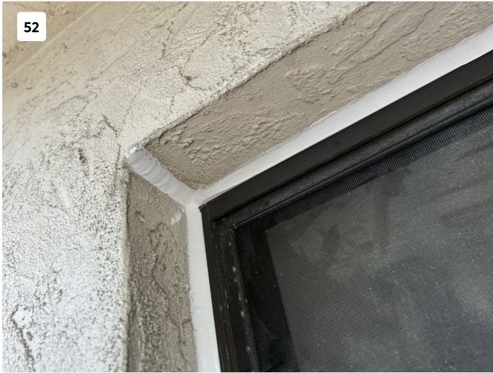
New window opening sealant.
