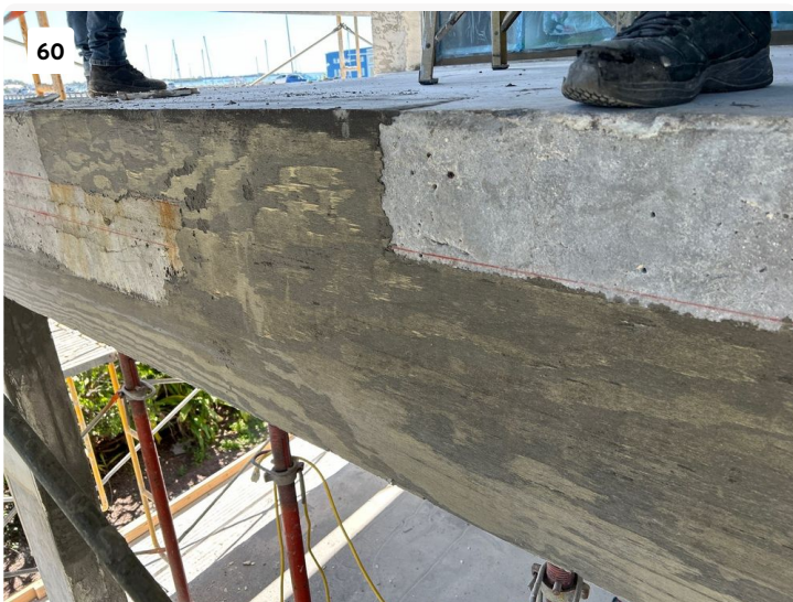
Balcony concrete repair.
