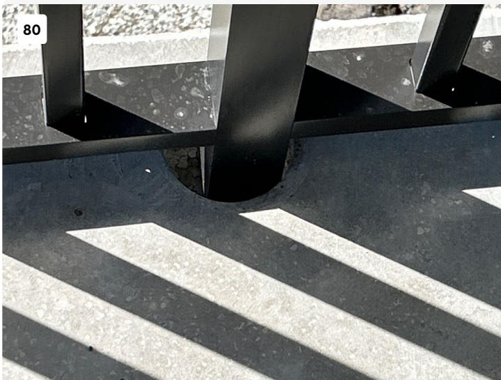
New rail post fitting in progress.
