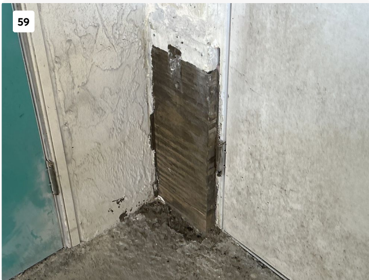
Concrete repair in garage.
