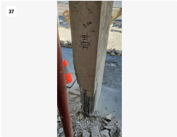
Garage column concrete repair in progress.
